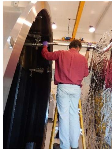
*Figure 14: Removal of Rear Shroud*
